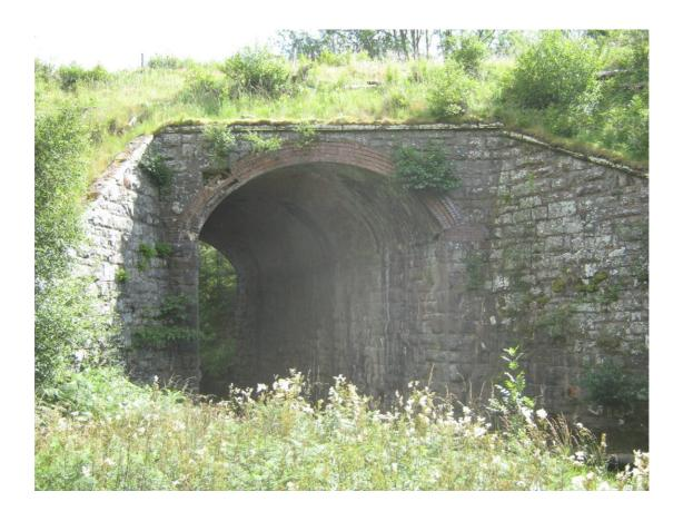
"A skew-arched bridge, carrying the former Mid-Wales Railway formation (nprn 303234) across the Afon Marteg some 700m east of Abermarteg. Constructed of coursed stone blocks with brick barrel-vault, the bridge is some 18m long and the span is about 9m."
